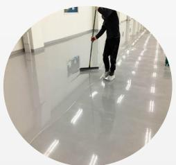
STEP 2. Pour the mixed paint on the floor and spread it evenly using a rake or squeegee..
