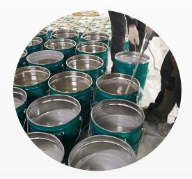
STEP 1. Mix base and hardener for 2-3 minutes using the electric stirrer.
