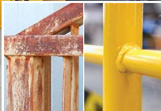
After applying the urethane universal primer
